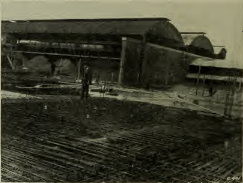
PART OF REVIVIFYING FLOOR, SHOWING MESH REINFORCEMENT.
